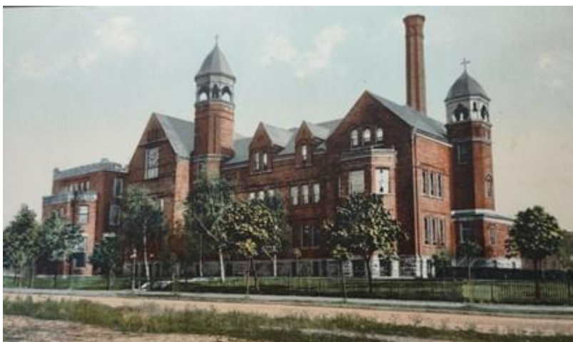
A view of the early Villa complex at West Eighth and Liberty streets prior to additions. Note the vacant land on the north side.
