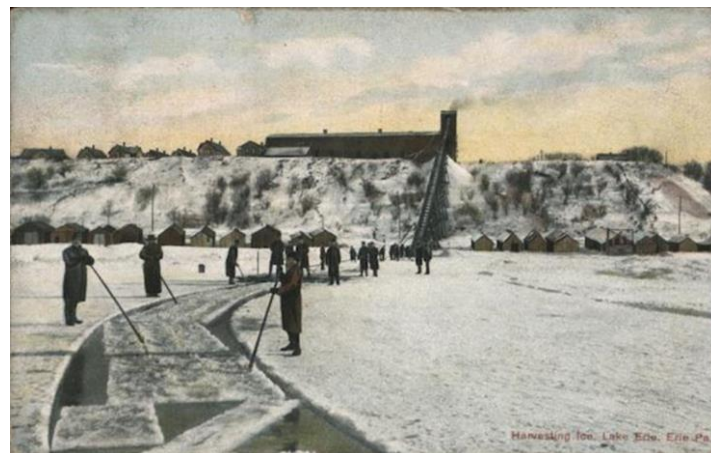
A typical bayside icehouse included a lifting conveyor that carried blocks of ice up and into a storage building.
